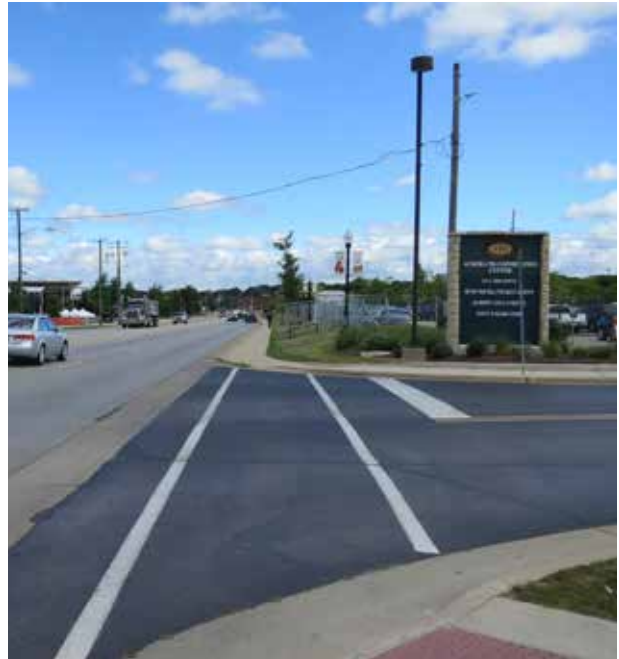
Large curb radii allow for easier turning movements for buses, but they result in a lengthened crossing distance for pedestrians and encourage drivers to take fast turns.
